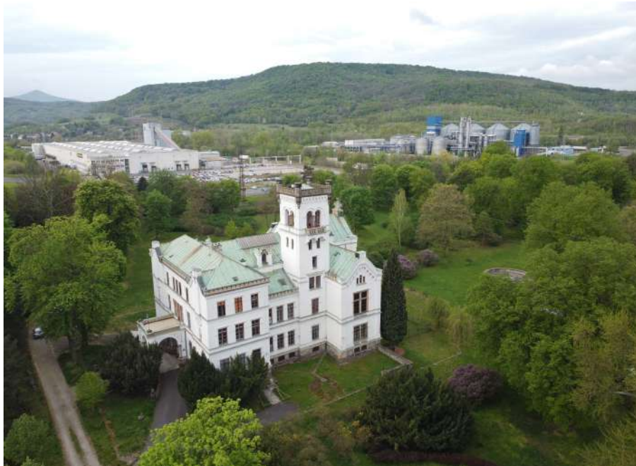
Trmice castle with industrial buildings in the background, source: PKÚ, s. p. photo archive
